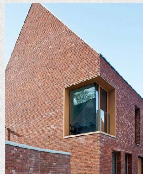
CORNER FEATURE WINDOWS + FRAMES COLOUR TO MATCH COLOURS FROM SELECTED COLOUR PALETTE
