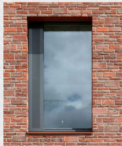
BRICKWORK + DEEP REVELS + VENTILATION PANELS + FRAMES COLOUR TO MATCH COLOURS FROM SELECTED COLOUR PALETTE
