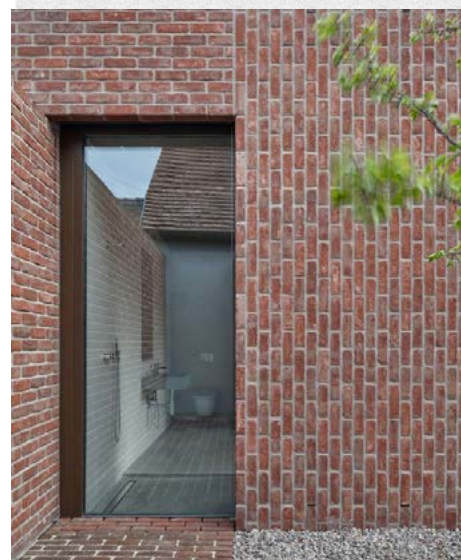
DIRECTIONAL BRICKWORK PANELS
