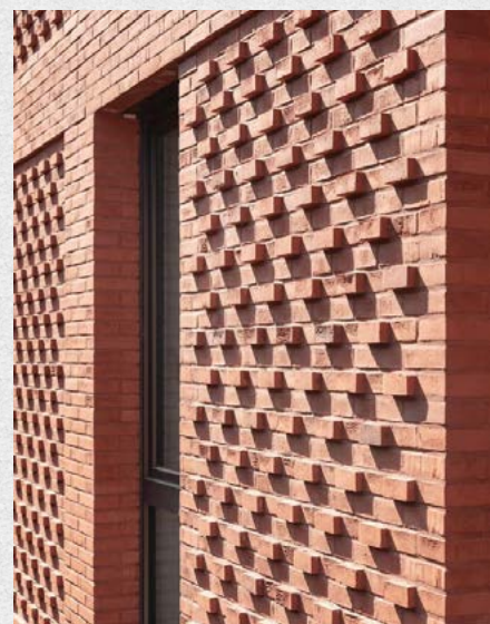
PROJECTING BRICK HEADERS PANELS
