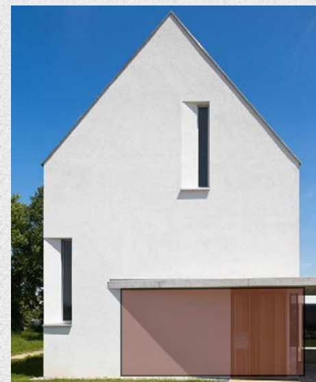
RENDER + SPLAYED WINDOW REVEALS + INDIVIDUAL COLOUR RECESSED ENTRANCES WITH COLOURS FROM SELECTED COLOUR PALETTE
