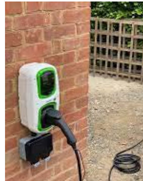
PV PANELS FOR SOLAR GAIN AND RENEWABLE ENERGY SOURCE & ELECTRIC VEHICLE-READY CHARGING POINTS
