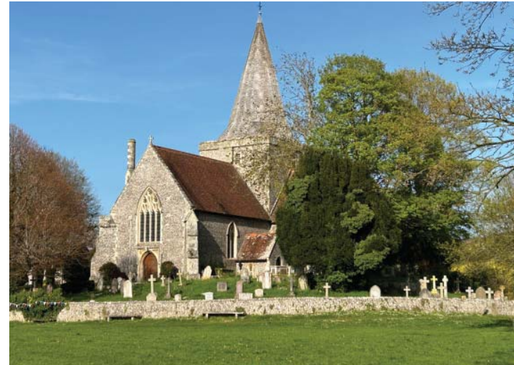
The church is the most prominent building to use flint, of which there are many examples.
