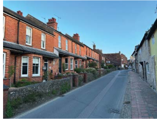
View B looking south down North Street with the site concealed behind the (left) terrace.
