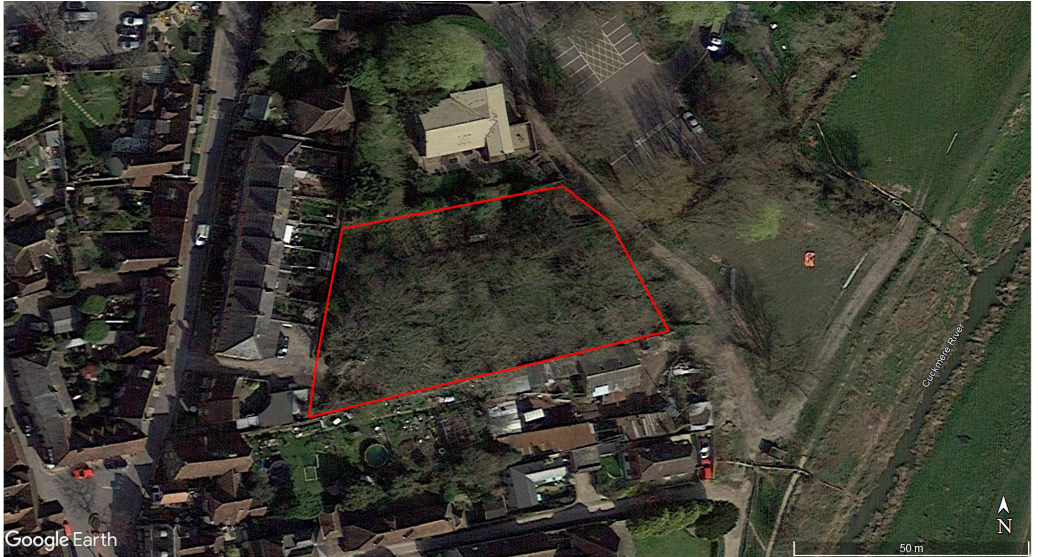
13.0 Figure No. 01 – Site Aerial
